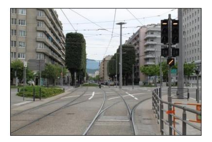
The railway signalling no longer manages converged routes, but still manages conflicting ones: the command of the railway needle and its security. This new managing solution permits a smoother global functioning and a bigger reactivity. Signalling communication with the driver is now simplified.
